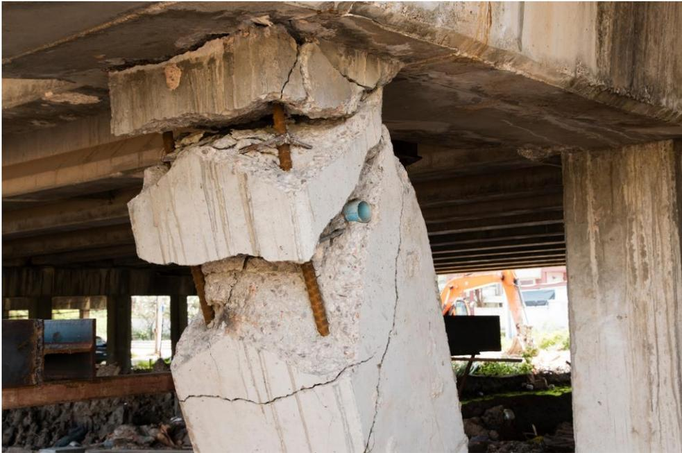
Cracking in concrete is a complete or incomplete separation of either concrete or masonry into two or more parts produced by breaking or fracturing (ACI Concrete Terminology)
